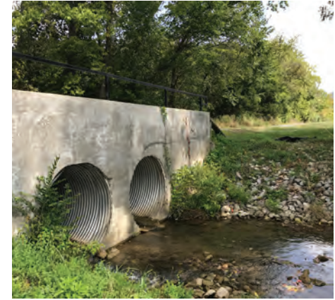
Bridge culvert over Town Run
