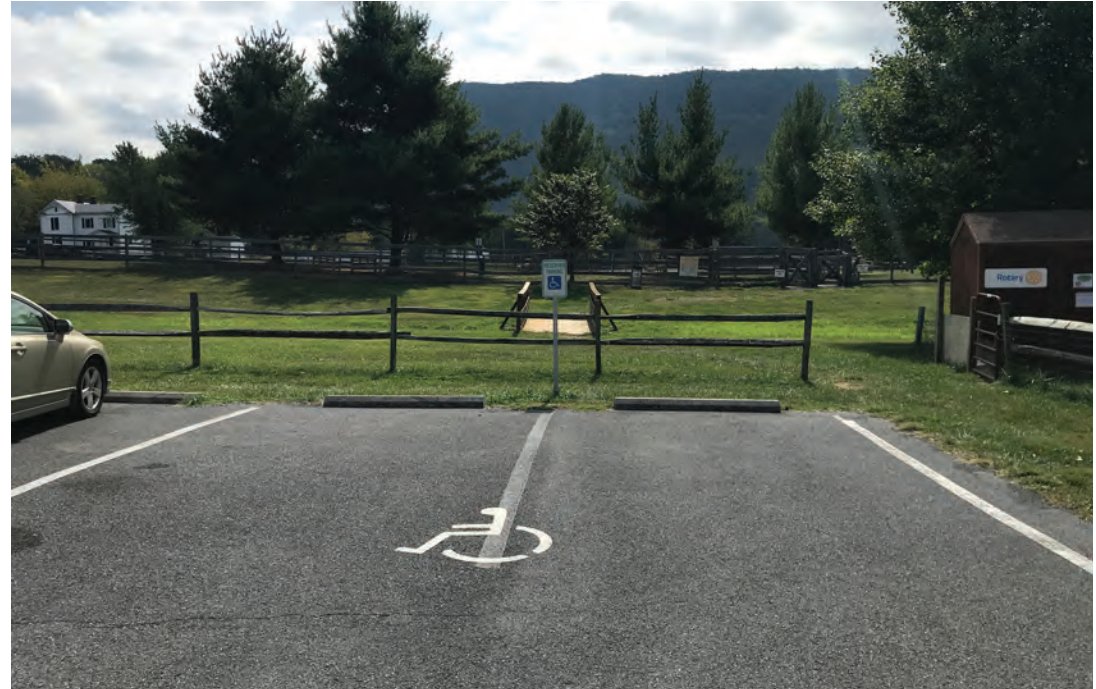
ADA Accessible parking at Town Park in one of the asphalt paved parking lots, an accessible route is needed to tie parking spaces to park features
