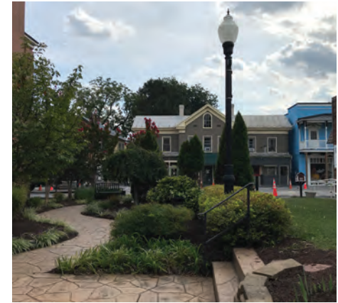
Stamped concrete path and steps
