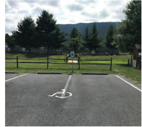
Accessible parking not clearly marked
