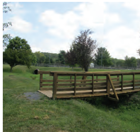
Pedestrian bridges not ADA accessible
