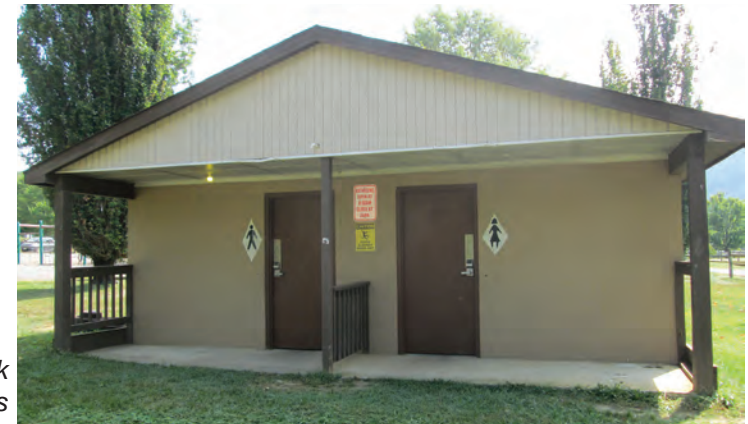
Town Park permanent restrooms
