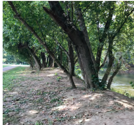
Eroded river bank lacking ground cover
