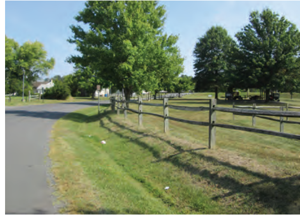
Drainage swale along Park Road
