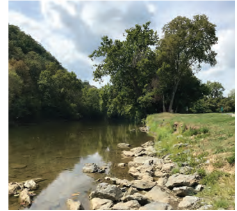
Rip-rap along banks at the boat launch
