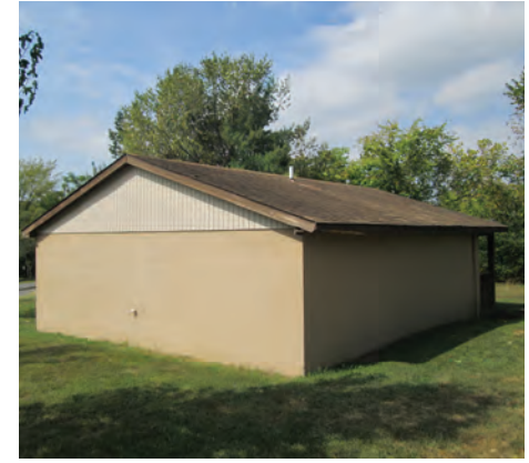
Entrance to restroom obscured
