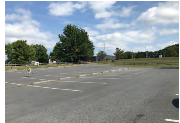
Lack of shade trees at parking lot with 40 spaces
