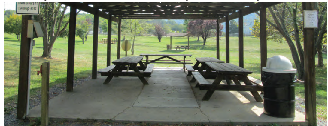
Shelter does not meet ADA standards; water pump and electric available at Kiwanis Shelter
