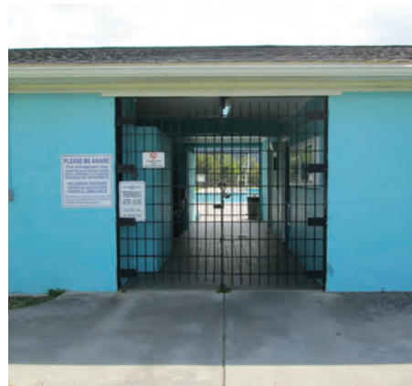
Entrance to pool house
