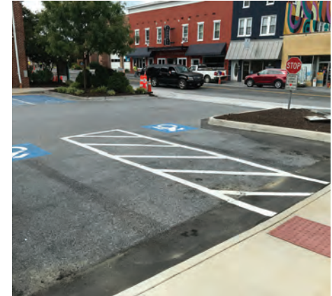
ADA accessible parking
