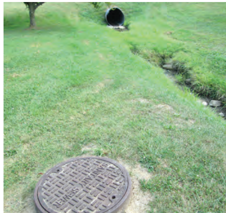
Sanitary sewer near drainage swale
