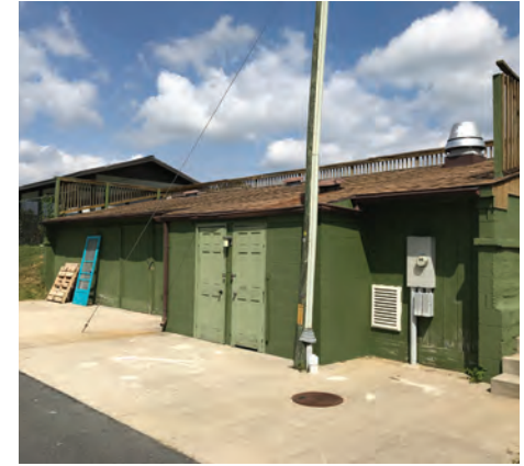
Pump house and maintenance area
