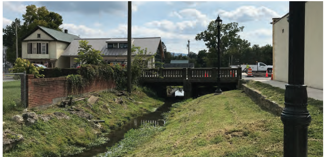
Consider future expansion to widen concrete sidewalk to better accommodate bicycles and other multimodal users
