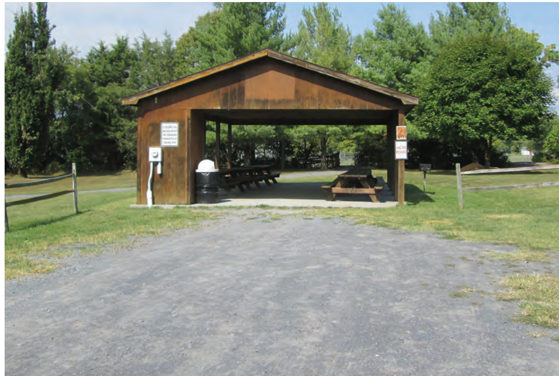
Town Park park shelter with gravel parking and access drive
