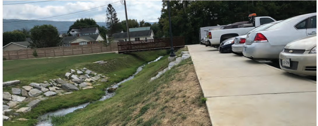
Strasburg Square on the left, the Town Hall parking lot and sidewalk on the right
