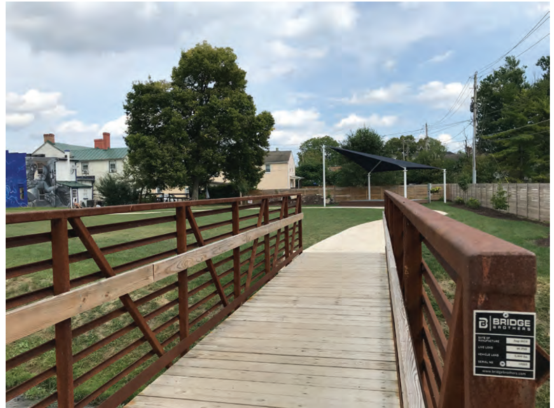
Figure 12- Pedestrian bridge from Town Hall to Strasburg Square, looking toward the sail-covered stage
