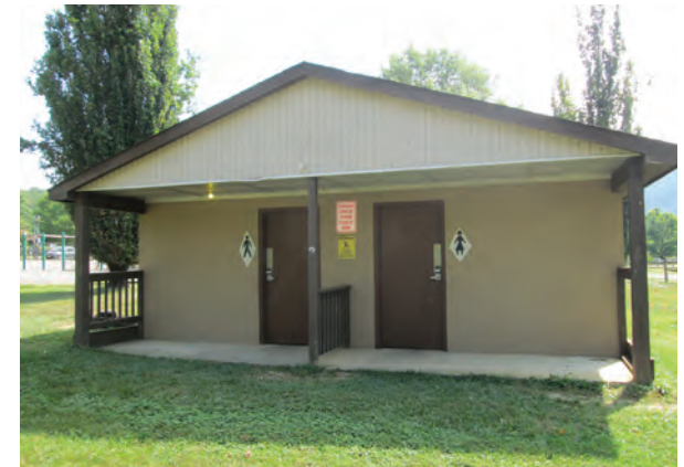
No accessible route to restroom facilities
